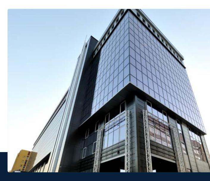
Pilkington Suncool® 30/16 Pro T offers the best protection from the solar radiation, regarding both light and heat. It finds its best use in large-area façades and horizontal roof glazing. Due to an extremely low solar factor (19%) this product is especially effective when keeping solar heat gain under control is paramount.
