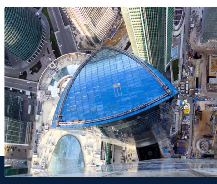
Pilkington Suncool®-R Blue 50/25 Pro T features a shiny blue appearance. Due to the unique magnetron coating technology it lets in neutral light inside the building without any colour distorsion. High light transmittance and selectivity of this product allow to get a comfortable inner environment with a coloured exteriour.
